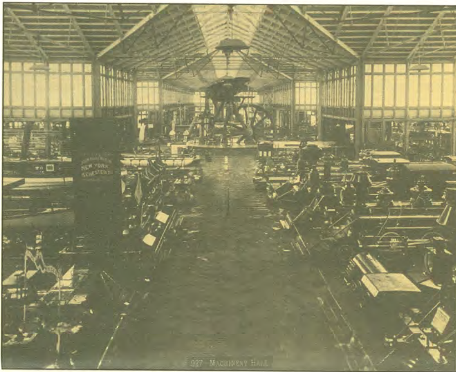
The great Corliss Centennial steam engine (under the transept in the center of the aisle), 43-foot high, 700 tons, generating 1,400 horsepower — in its day the most powerful engine ever built — powered all of the operating machinery in the 14-acre Machinery Hall during the "International Exhibition of 1876," Fairmount Park, Philadelphia, between May 10 and November 10, 1876. (Photo #927, Centennial Photo Collection, Print & Pictures Department, Free Library of Philadelphia. From the collection of Robert Cotner.)
