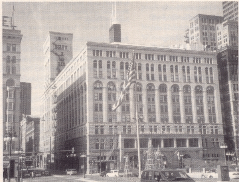
"The culmination of Louis' masonry 'period,'" the Auditorium Building (1887), Congress St. and Michigan Ave., "with its immense mass of ten stories, its tower, weighing thirty million pounds, equivalent to twenty stories — a tower of solid masonry carried on a 'floating' foundation; a great raft 67 by 100 feet." ( Autobiography , pp. 303, 309)
